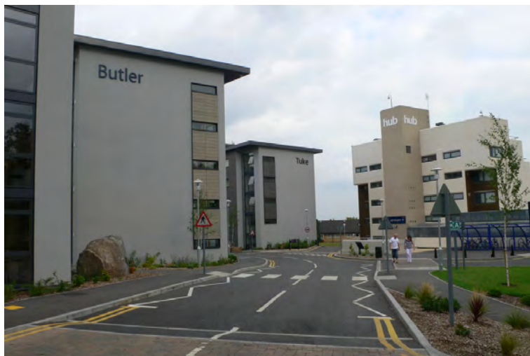
Figure 4: Hostels building for the participant (Butler and Tuke), the Hub building is the information centre for check-in/out, do laundry, buy meals etc.
