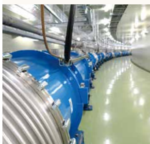
Superconducting magnets in the J-PARC Neutrino Experimental Facility
